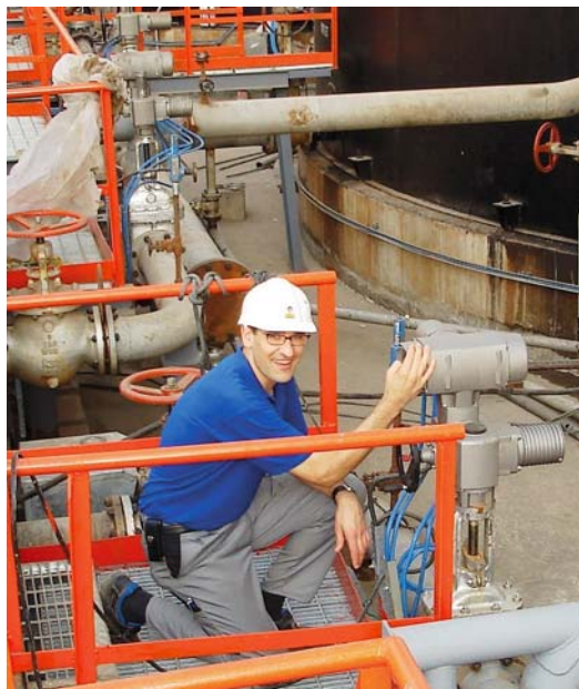
AUMA actuator with Modbus-RTU interface automating multiturn-turn valve
