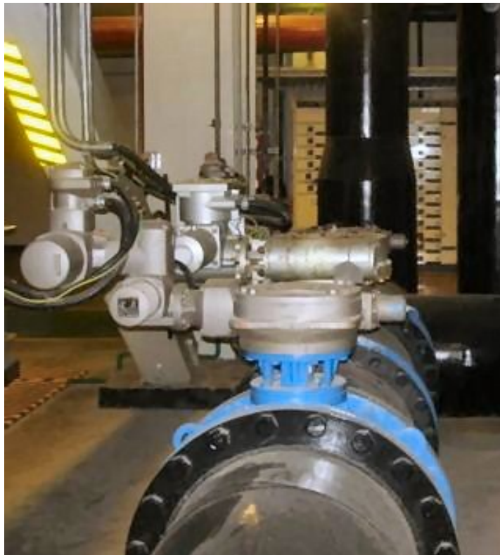
AUMA actuator with PROFIBUS DP interface automating part-turn valve
